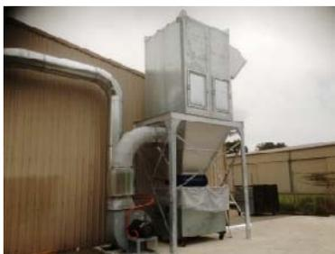
The unit is also supplied with a Porex Variable speed Drive Controller or VSD. The VSD is supplied with a pressure transducer that will sense and automatically turn the power consumption of the fan motor down when one or more of the machines is not in use. **This equates to big savings on power consumption.** Lambert Kitchens is very happy with the performance of the unit, the ducting & the service they received from Ezi-Duct and Porex Environmental Engineering.
